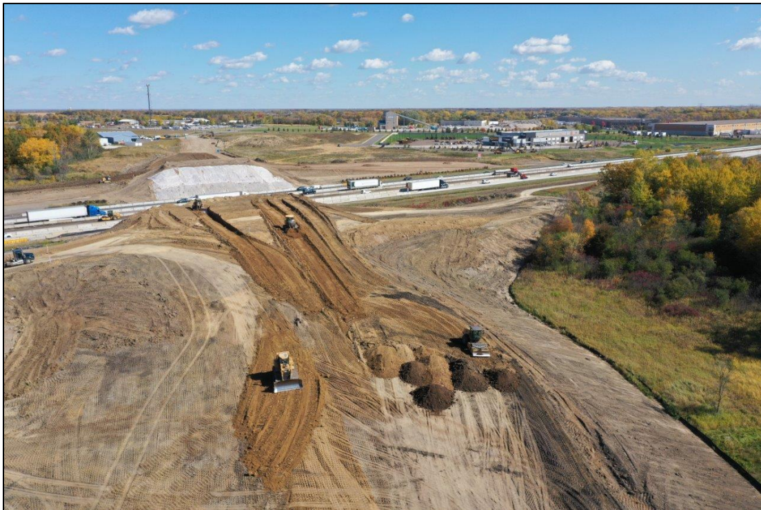
A view of the Dayton Parkway embankment grading west of I-94 looking to the east
