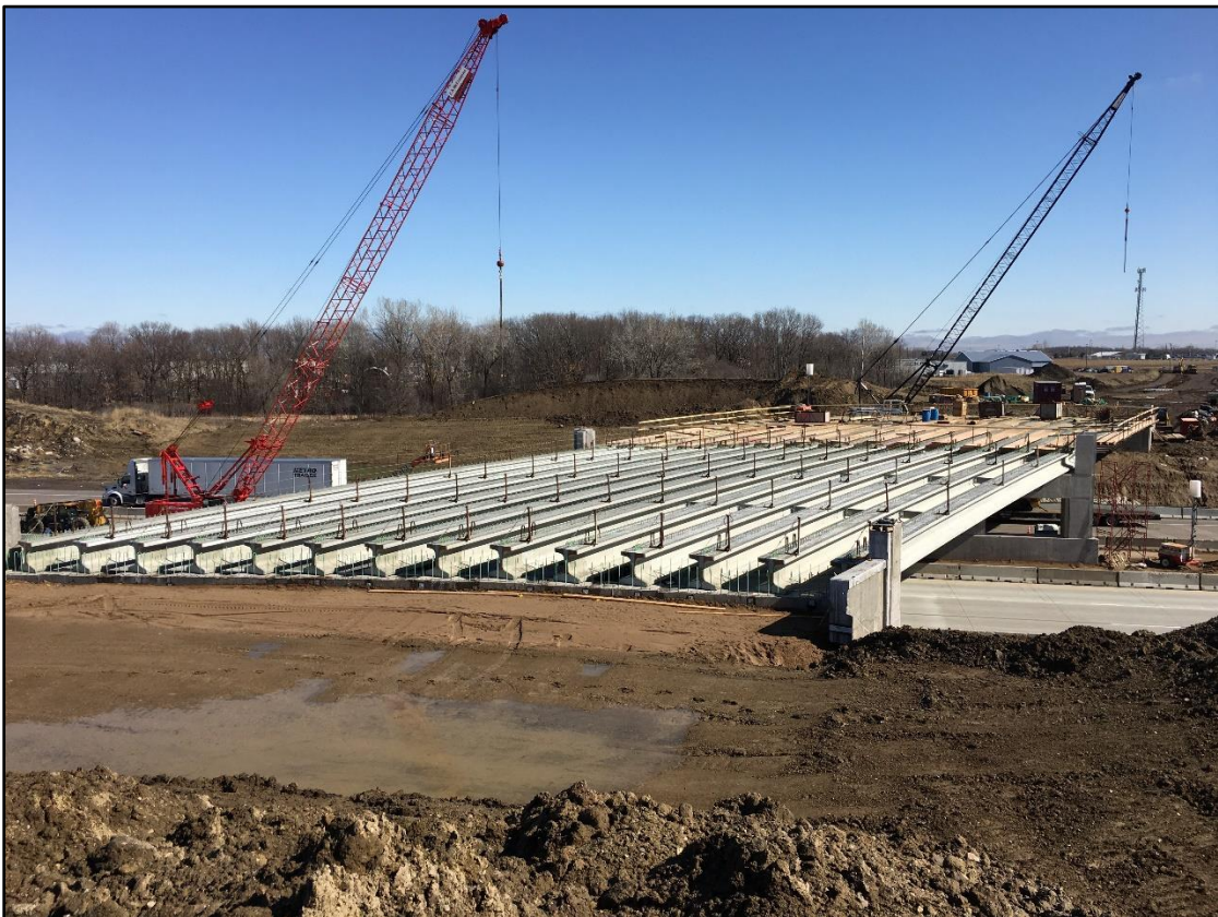
A view of the Dayton Parkway bridge beams over I-94 from the west abutment looking to the east.
