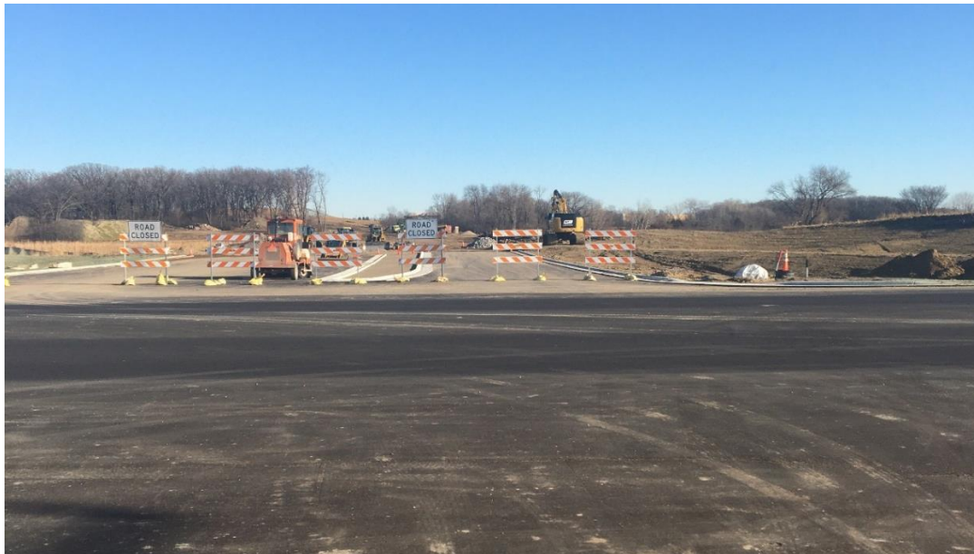
A view looking down the future Dayton Parkway from the Brockton Lane intersection.
